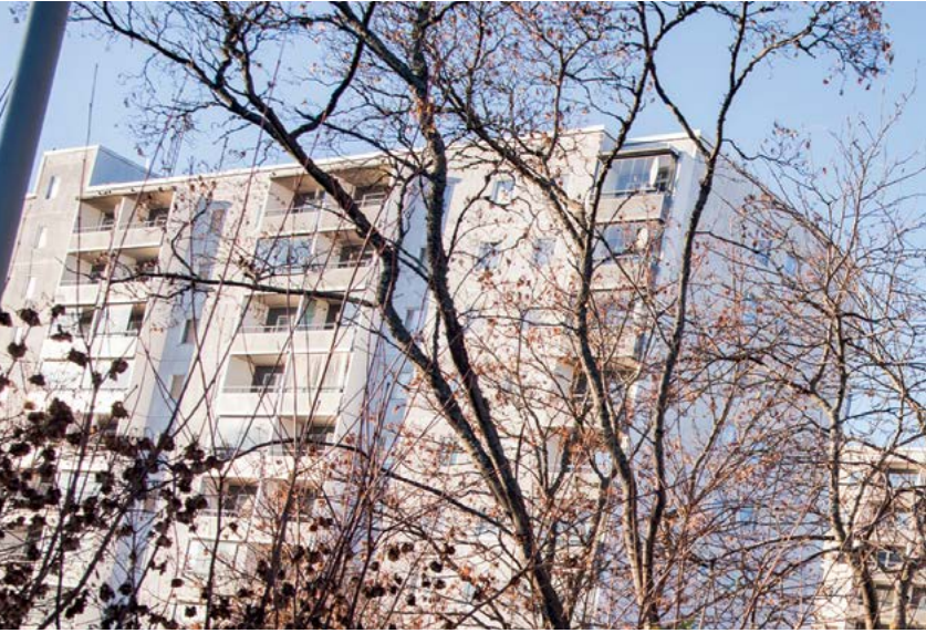
Tower blocks in Husby
